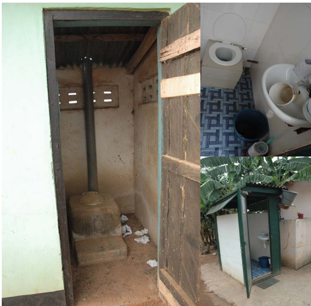
Figure 44: The old VIP latrine still being used by Samuel's father (left) and the new MFBF toilet facility (right-below) with an enlarged view of the sink and toilet (right-above)
