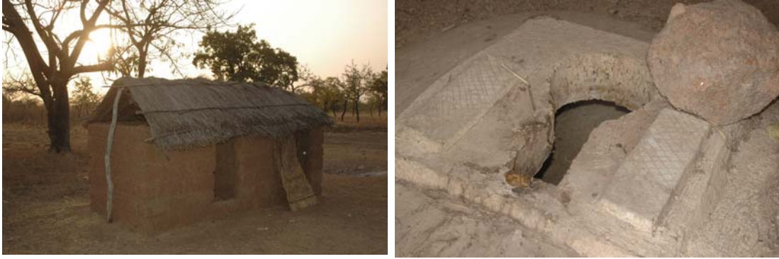
Figure 38: One of the latrines in the Suburi Village (left) and the DA-provided concrete slab with cover inside (right)
