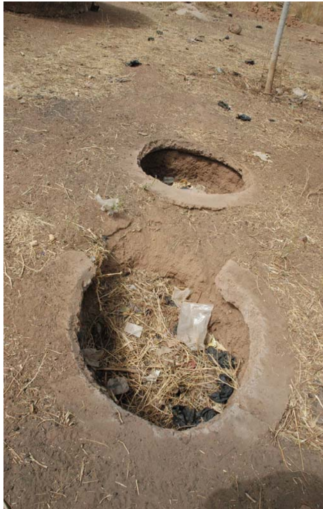
Figure 28: Partially dug pits that were never finished or previously collapsed were found throughout Challam
