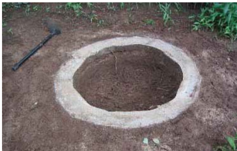
Figure 13: Arborloo Ring Beam (WaterAid)
